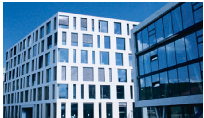
New-built facilities of Brugg Cables in Switzerland, including the rooms of the Brugg Cables Academy
