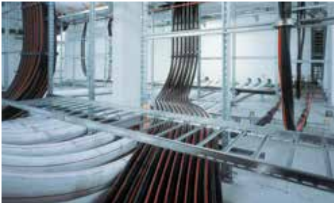
Medium-voltage cables
