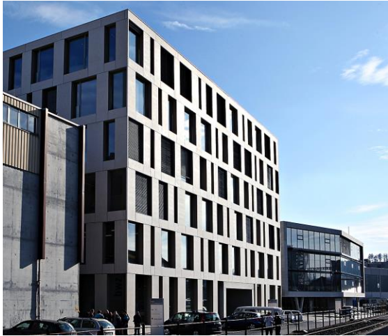
Caption: Building exterior location at Brugg
